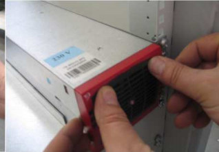
(3) Close the cover and latch the module in place If too hard redo step (2)
